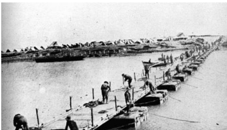
Fig.2: Pontoon bridge built by 3 rd Fd Coy, January 1915, at this time located at El Kantara (RAEAWA Archive).
