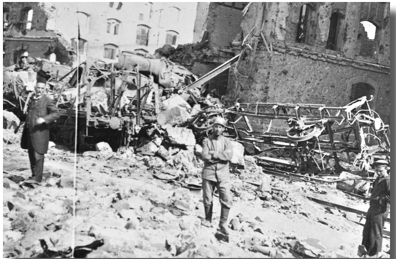
Figure 18: Wrecked rolling stock among rubble, possibly the Tul Keram railway station (see Fig.17). At centre and right are an Asien-Korps soldier and a sailor. Source: Fletcher collection.
