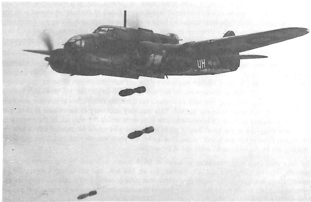
Two 500-lb bombs leaving the bomb bay of Beaufort A9-427 of No 100 Squadron. A 250-lb bomb with streamer has dropped from the wing bomb carrier.
