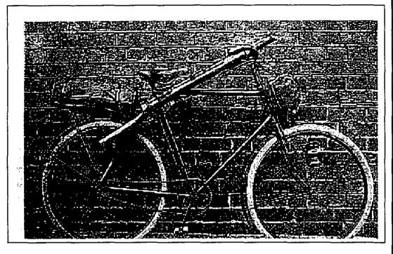
A rugged and apparently very reliable, single gear, steel frame cycle, the Mk. I was fitted with carrying clips for the .303 Magazine Lee Enfield rifle, as well as carrying frames and straps at front and rear for personal equipment.<sup>88</sup>
