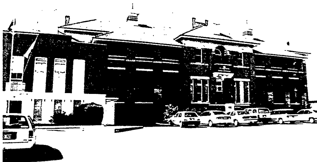
Artillery Barracks, Fremantle showing wing occupied by Army Museum
