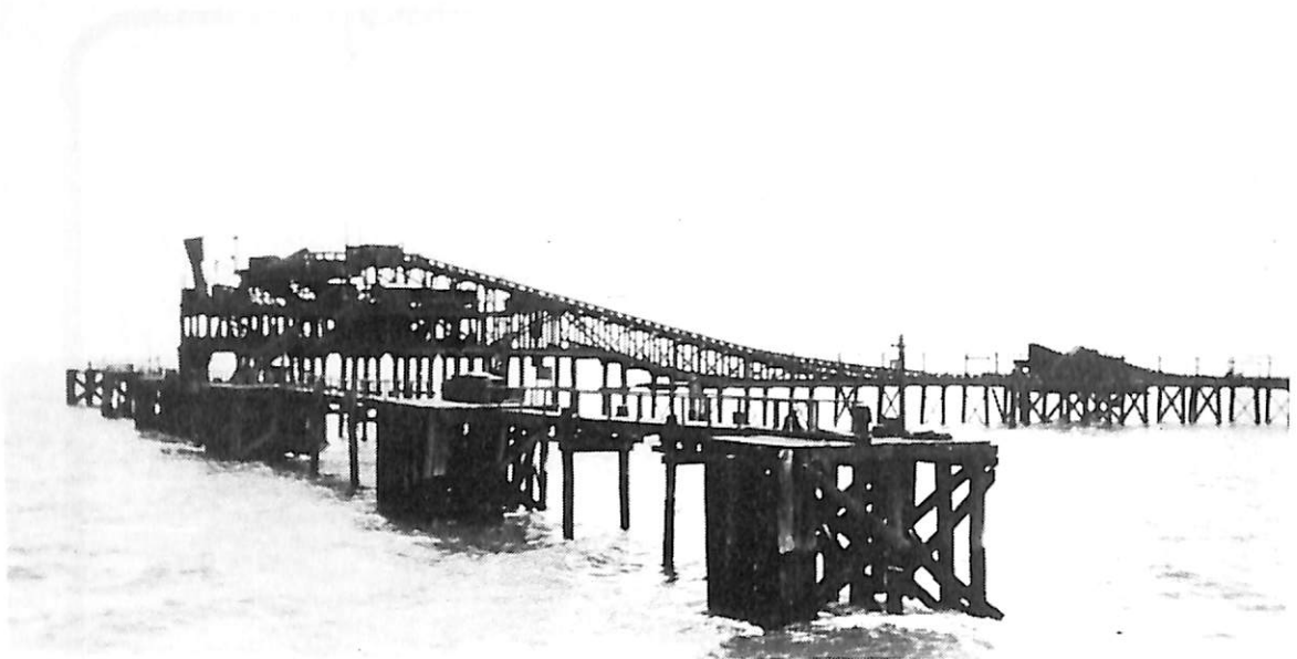
Whyalla's ore jetty, the reason for the town's industrial and strategic importance (South Australian Archives).
