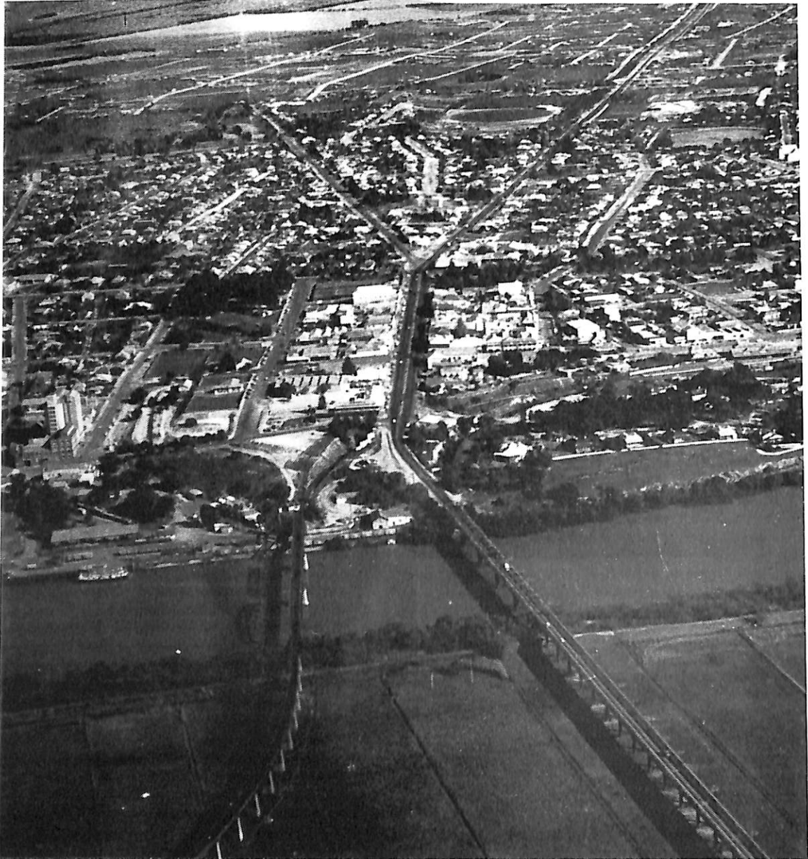
The two bridges and the town of Murray Bridge, looking west.
