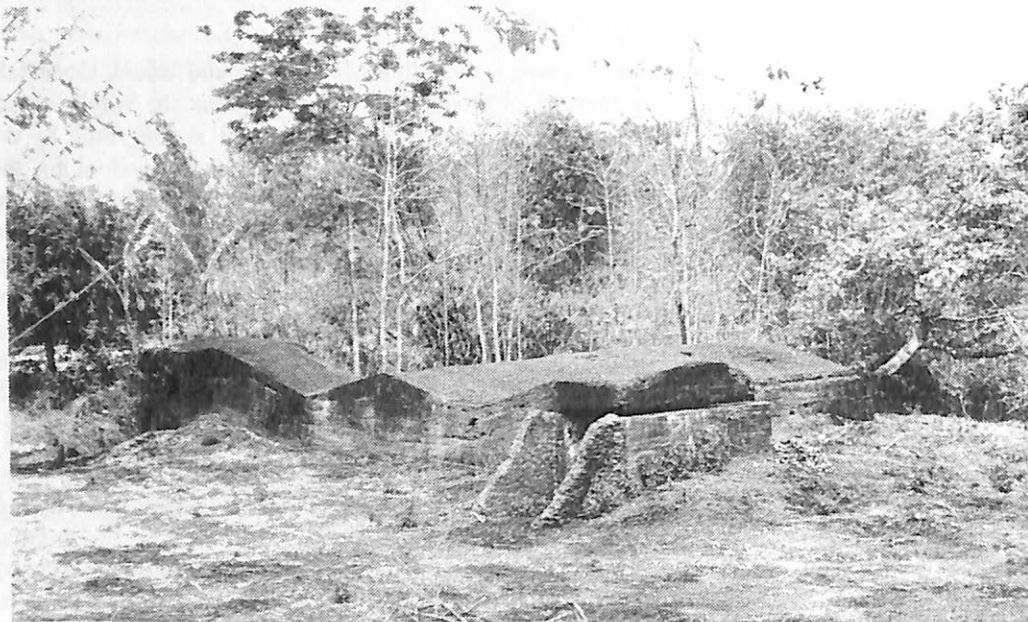
Japanese bunkers at Macopa on the road to Bantimurung, Kapupaten of Maros, South Sulawesi.
